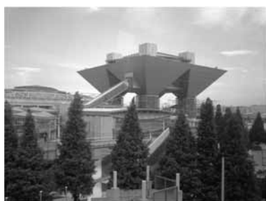
Figure 4. The Tokyo Big Sight Building 7 , The main press center of 2020 Games
